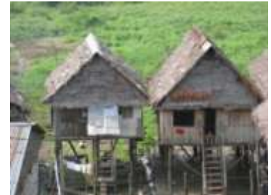
In the Amazon River basin, people build houses on stilts to protect themselves from floods.
