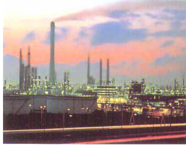
Installation of power plants
